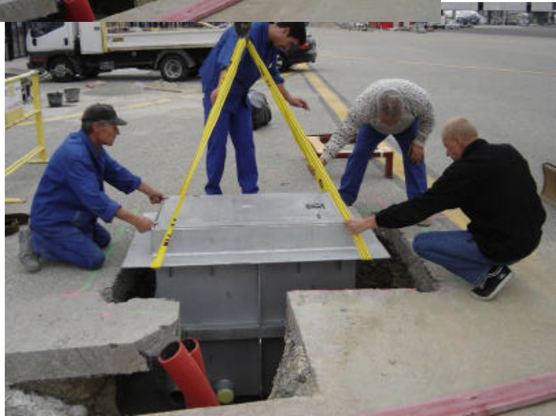
Positioning of Pit using slings around top angles.
